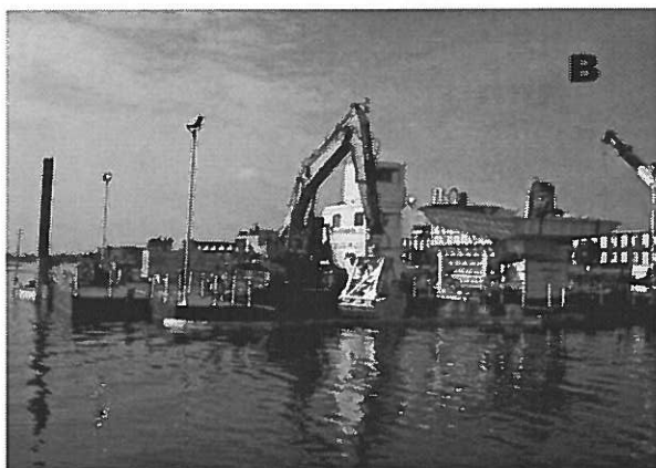
Note: A = Cable Arm Corp. dredge (Source: Cable Arm, Corp.) B = Bean Company Horizontal Profiling Grab (HPG) dredge, New Bedford Harbor Site (Source: Barbara Bergen, U.S. EPA)
